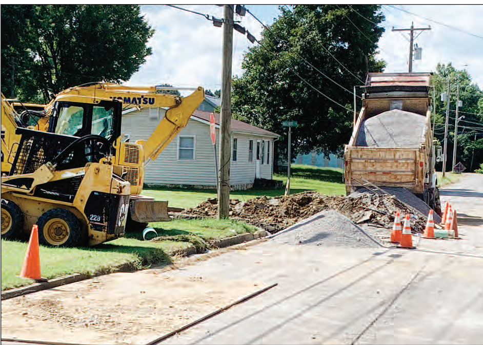
THE CRITTENDEN PRESS Work this summer on Marion's sewer system overhaul has concentrated on digging up and replacing old lines, but work transitioned this week to slip-lining to upgrade lines.
